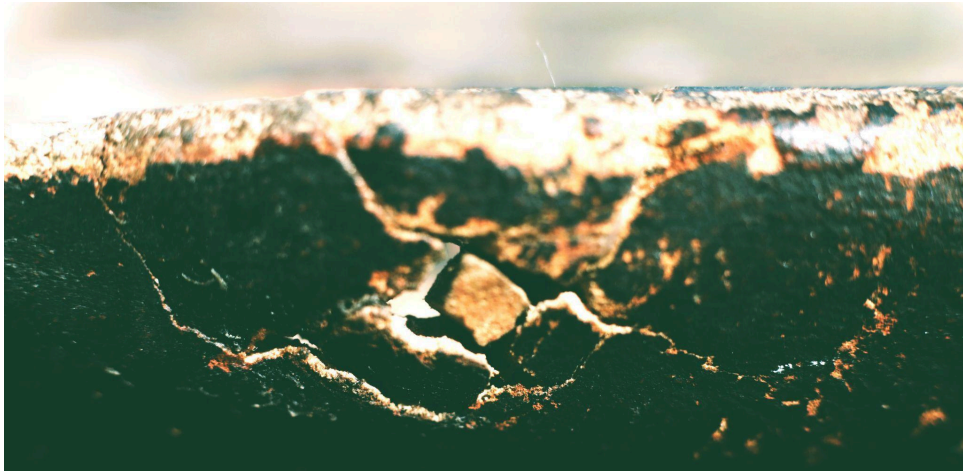
Figure 6: Reappeared damage on Bao board (Photograph by Jack Alexandroff, 2025)
